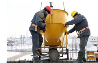
Concrete Construction services
