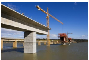
Road and bridge construction
